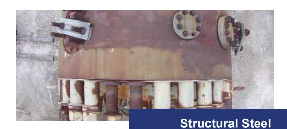
Missing or loose bolting is one of the most common discrepencies found during structural inspections. While aerial inspections cannot verify bolt or stud torquing, it can pinpoint installation discrepancies on new and existing structures.
